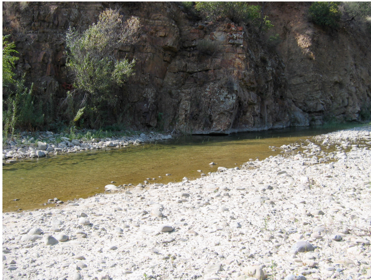
Bedrock scour pool SC1 adjacent to Water Canyon Campsite.
