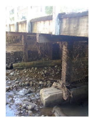
This older bridge contains wood supports on concrete footings that occur within the stream channel. The footings and supports are significant debris blockage features that increase the likelihood of failure and/or adjacent flooding. Removal of this bridge and adjacent pipe and wire revetment and installation of a wide-span bridge would enhance stream habitat, sediment transport, and reduce flooding potential.
