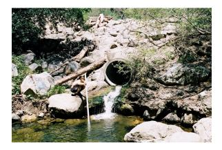
This County operated concrete and boulder debris basin dam conveys flows low flower through a smooth concrete culvert with a length of 68 feet 8 inches and slope of
