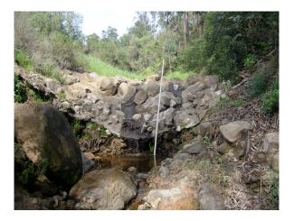
This 10-foot tall boulder and concrete dam occurs approximately 100 feet upstream of the Chelham Creek confluence. The dam is completely filled in with sediment and conveys all flows over the dam and downstream face. The usefulness of this dam should be determined and dam removal feasibility assessed.
