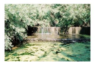
This concrete structure spans 41 feet across the stream channel and drops flows 3 feet onto a concrete apron that extends 12 feet downstream. This structure would prevent any upstream fish passage during low and moderate flow conditions. The structure could
