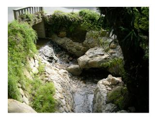
This concrete box culvert occurs on private property adjacent to Highway 192. A steep concrete apron occurs at the outlet of this culvert and drops flows 5 feet to the downstream substrate. This structure should be further assessed with landowner cooperation and removal and bridge installation considered.
