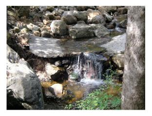
A concrete apron occurs approximately 150 feet upstream of the Coyote Creek confluence. This apron drops surface flows approximately 4 feet to a downstream pool with a depth of 2 feet. This structure does not appear to have a current use and may be associated with the nearby concrete chute on Coyote Creek just upstream from Chelham Creek. This obsolete structure should be further assessed and if feasible removed to allow ecological connectivity and improve potential future fish passage.
