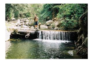
A 20-inch diameter pipeline crosses the creek with damaged concrete across the top. The height from the surface of the downstream pool to the top of the pipe and
