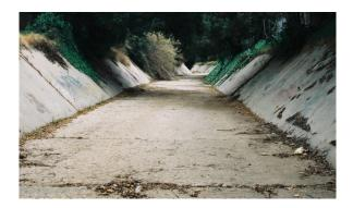
The second CALTRANS channel measures 0.27 mile. This concrete trapezoidal channel is similar to the downstream CALTRANS channel. A 2-foot drop occurs at the channel outlet. After this short jump upstream migrating steelhead would encounter
