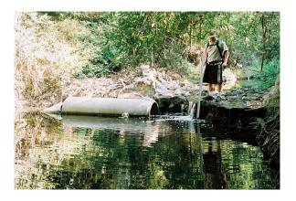
This small concrete and boulder grade control structure occurs near the 100-foot elevation and spans 17 feet across the creek. The old structure is in poor conditions with adjacent failed concrete culverts and bank erosion on river-right. During low stream
